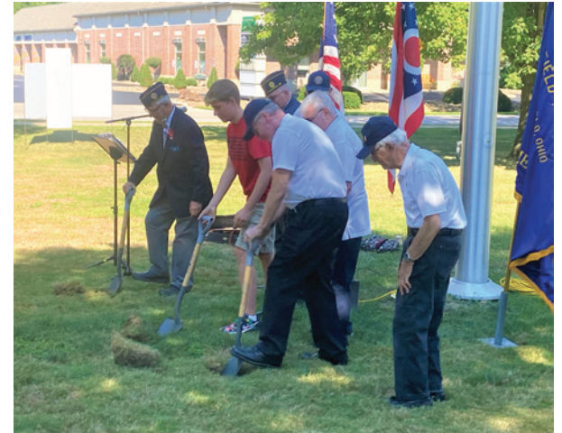
(left to right w/shovels) Post 177 Commander Kubitza, Scott Crawford, and Post Adjutant Chuck Coleman turn soil for the official ground breaking of the Canfield Veterans Plaza. (foreground right) Post 177 member, Frank Micchia.
